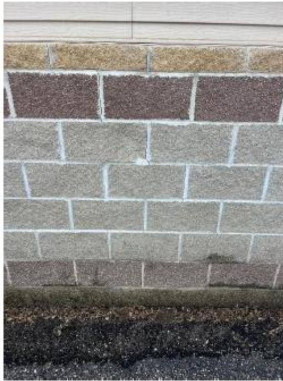
Photo #3: Cracks in veneer
