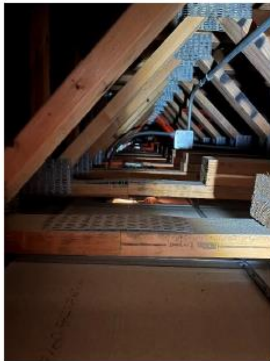
Photo #2: Bowing gusset plate
