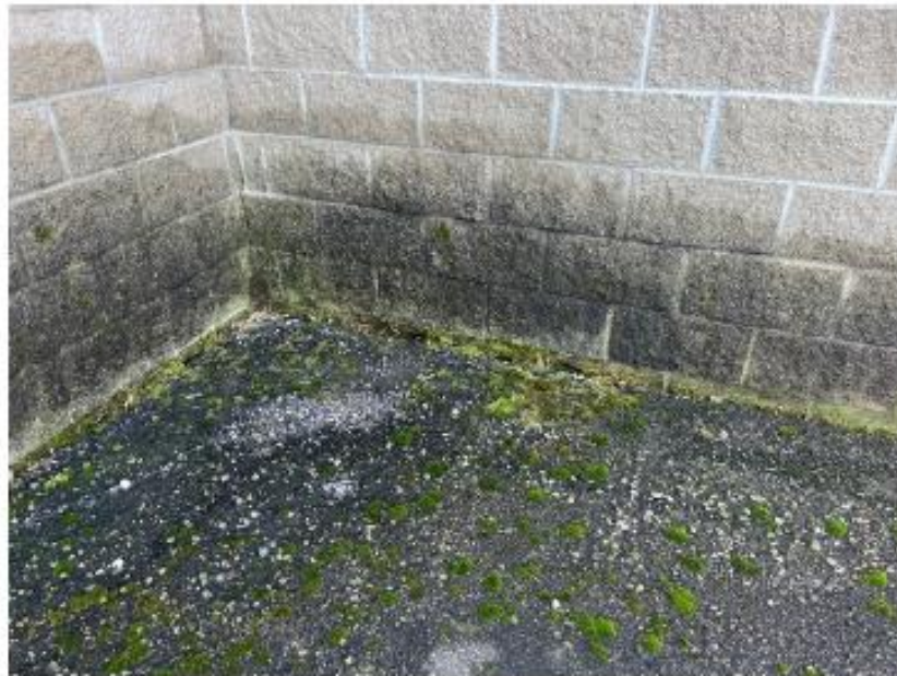
Photo #4: Deteriorated veneer
