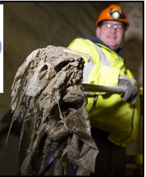
Wipes raked off a bar grate in a lift station in Eagan, MN.
