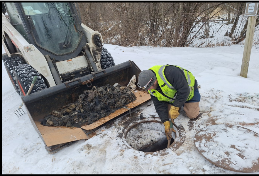
Frazee Public Works staff, Jesse Grossman, raking wipes off a bar grate.
